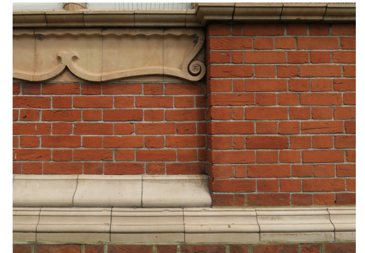
Venue 28 Brickwork Detail - Brick + Terracotta
