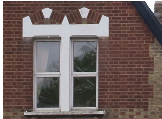
Housing, Beckenham Road, Brickwork Detail - Red + Yellow Brick
